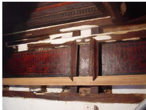
Consolidation of Horizontal Frames
