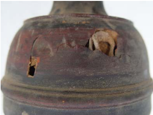
The Components appearing in sound condition from outside were found Hollow
