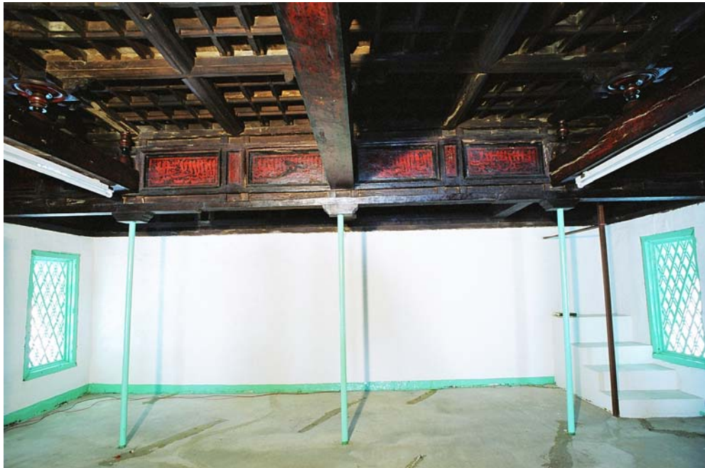
Iron Poles introduced during last Intervention
