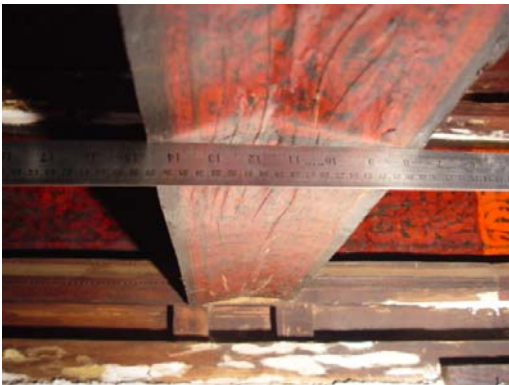
Different State of Deterioration of the Beams
