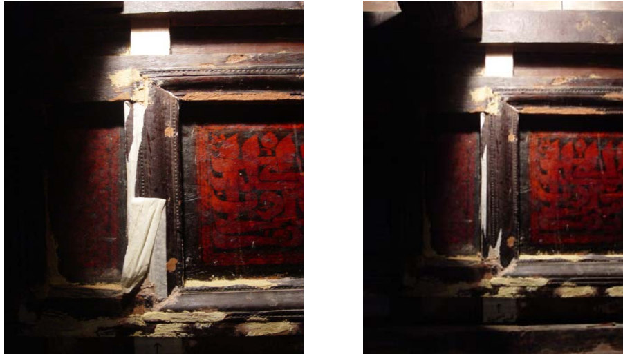
Consolidation of Vertical Frames
