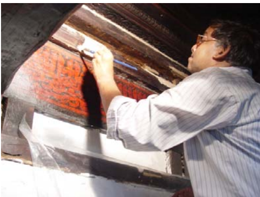
Consolidation of Horizontal Frames
