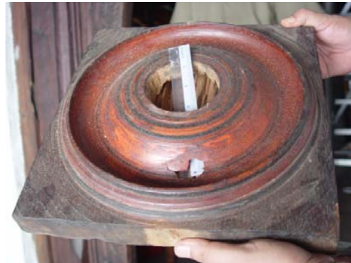
The Components appearing in sound condition from outside were found Hollow
