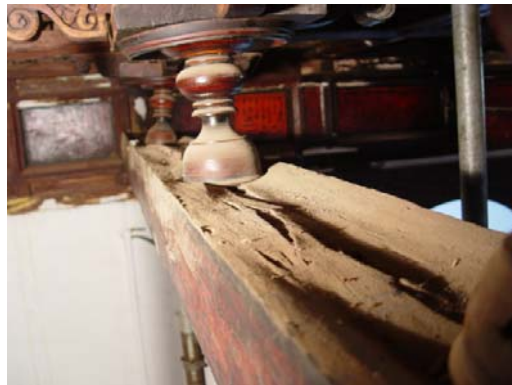
Different State of Deterioration of the Beams
